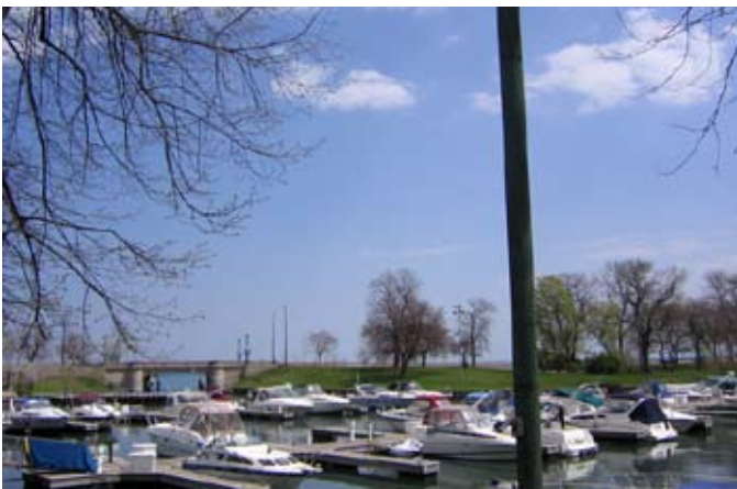
View of 59th Street Harbor with entrance under the South Lake Shore Drive roadway viaduct visible in the background
