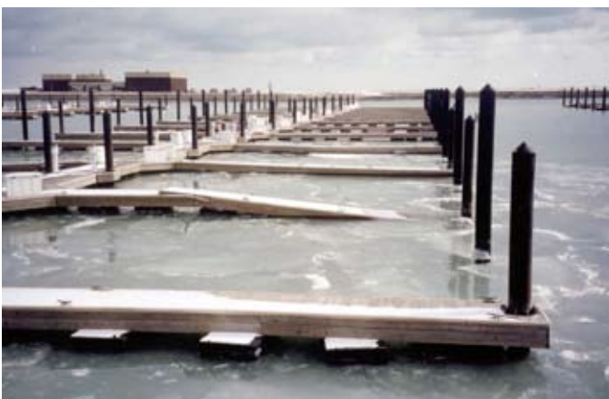
Ice damage to dockage at Burnham Harbor
