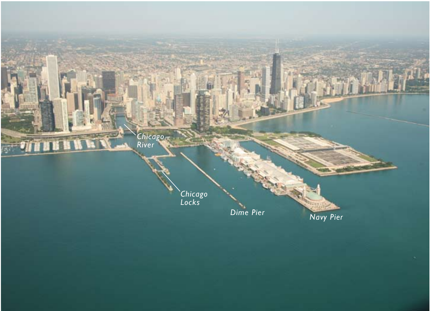
Current view of Dime Pier and Navy Pier
