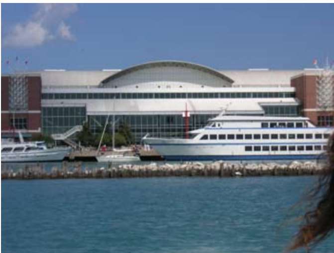
Excursion boats docking at Navy Pier (with dilapidated Dime Pier in foreground)
