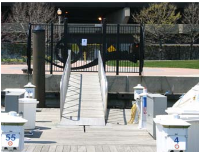
A combined security gate and accessible ramp at DuSable Harbor
